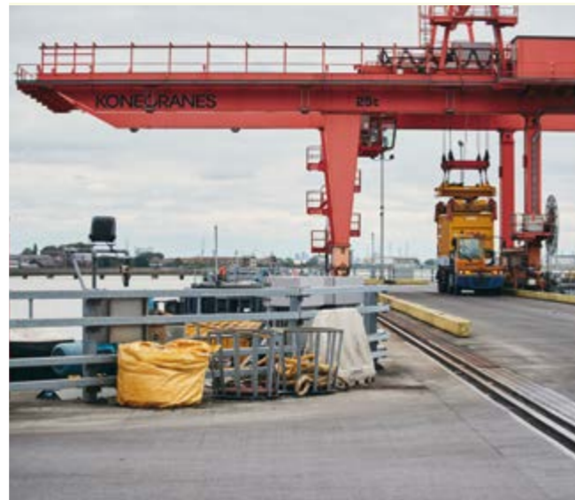
Jetty operations at the Riverside EFW facility.
