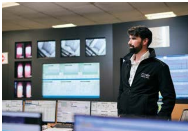
The central control room at our Riverside EfW facility is manned 24 hours a day, 365 days a year.
